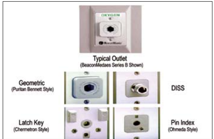
Figure 3 Medical gas and vacuum outlets Source: BeaconMedaes
